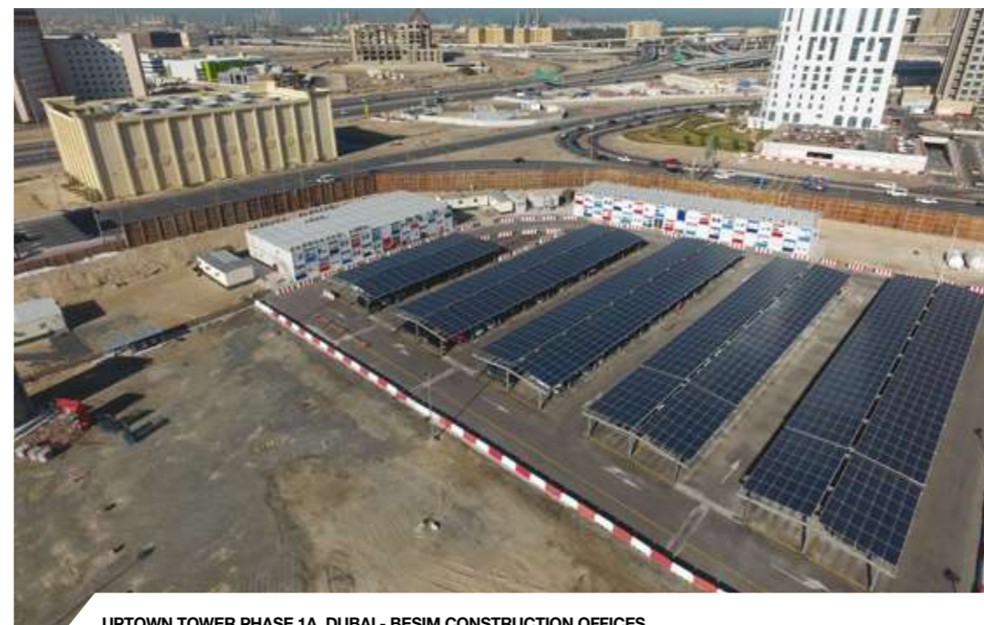
UPTOWN TOWER PHASE 1A, DUBAI - BESIM CONSTRUCTION OFFICES
