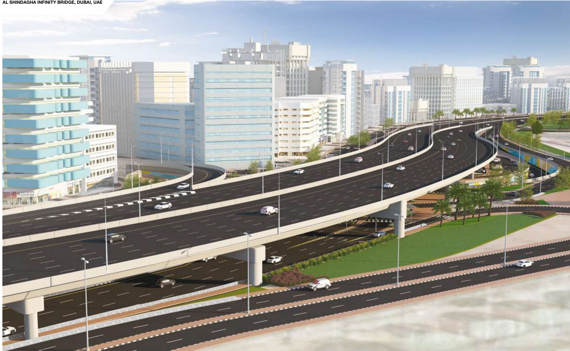
AL SHINDAGHA INFINITY BRIDGE, DUBAI, UAE
