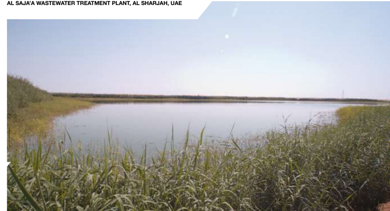
AL SAJA'A WASTEWATER TREATMENT PLANT, AL SHARJAH, UAE
